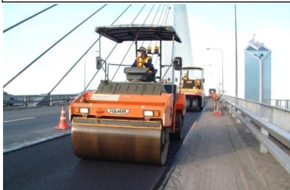
Rama 9 Bridge (Outbound) - EXAT
