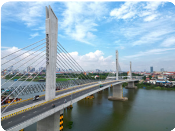
Russey Keo Bridge Project in Cambodia
