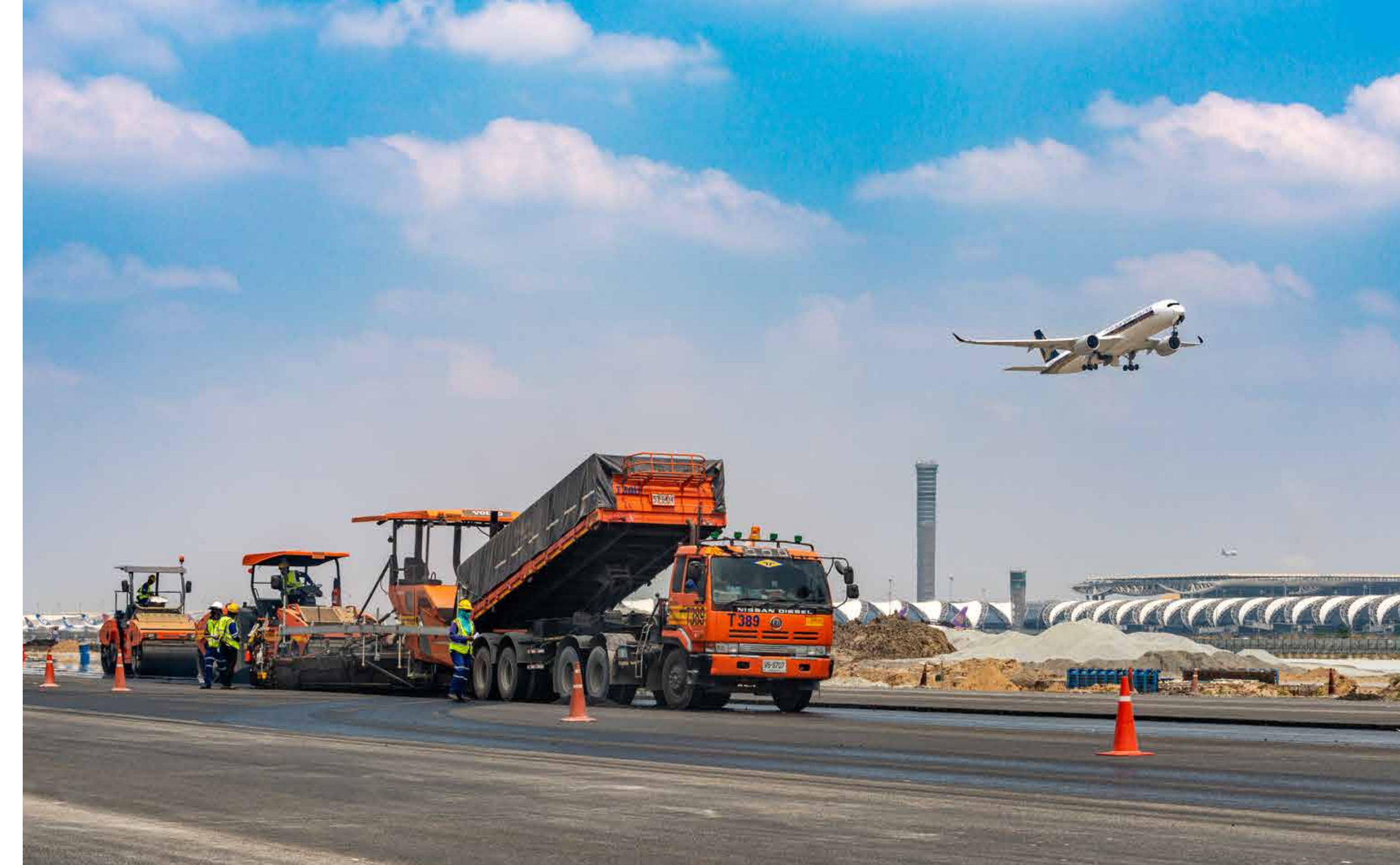
The 3 rd Runway Construction Suvarnabhumi International Airport
