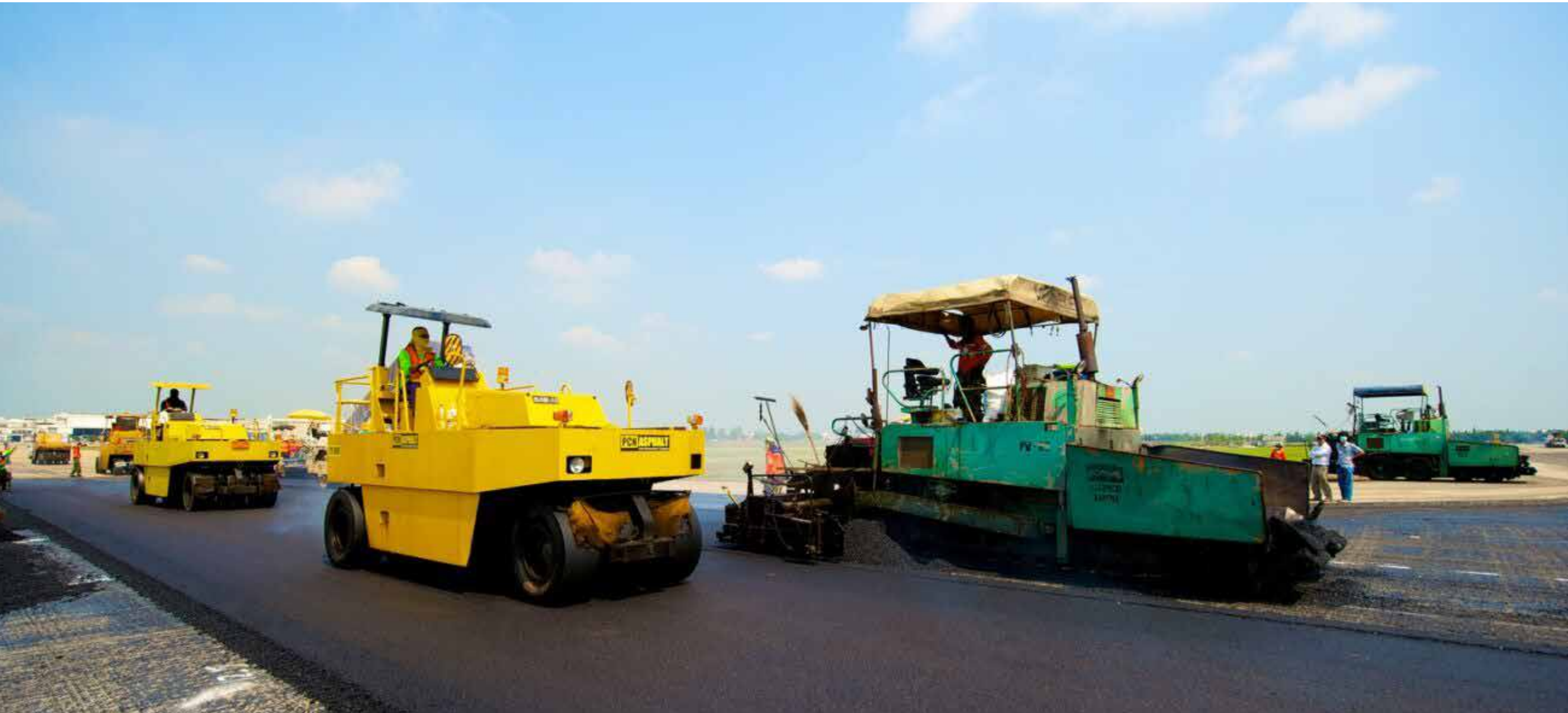
Runway and Taxiway Maintenance Don Muang International Airport
