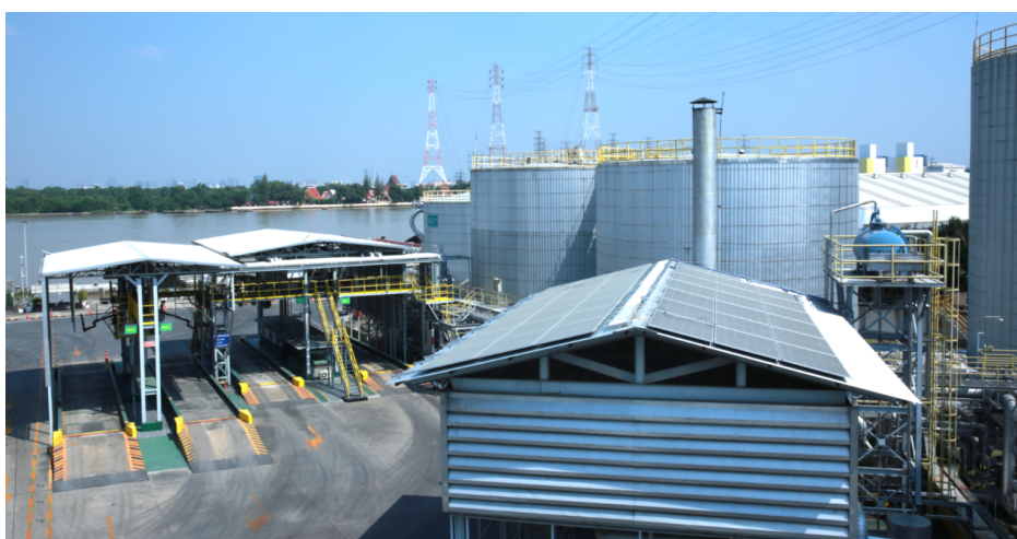
Solar Roof at Phra Pradaeng Plant
